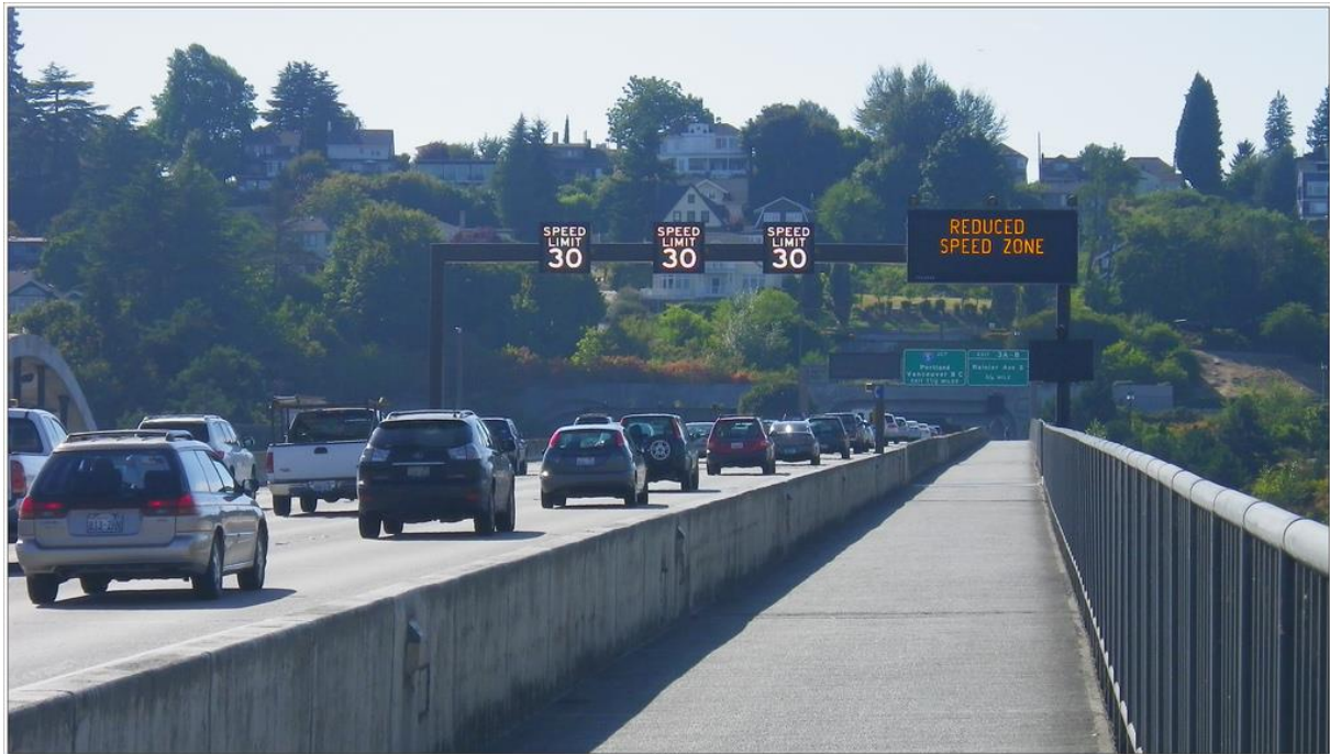
Figure 2: Typical VSL strategy implemented on a highway (Source: hdimagelib.com).
